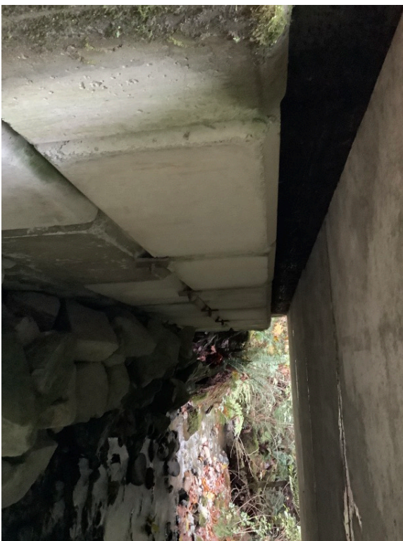
Right Bank Abutment when facing downstream
