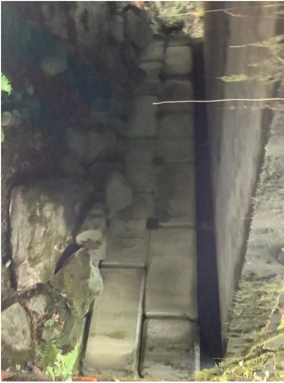
Left Bank Abutment when facing downstream
